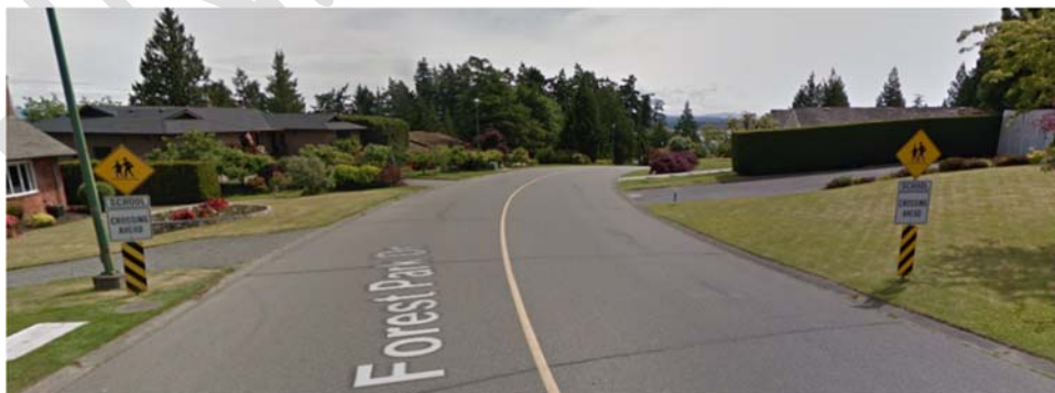
Non-standard ‘Crosswalk Ahead’ Signage 200m West of Crosswalk
