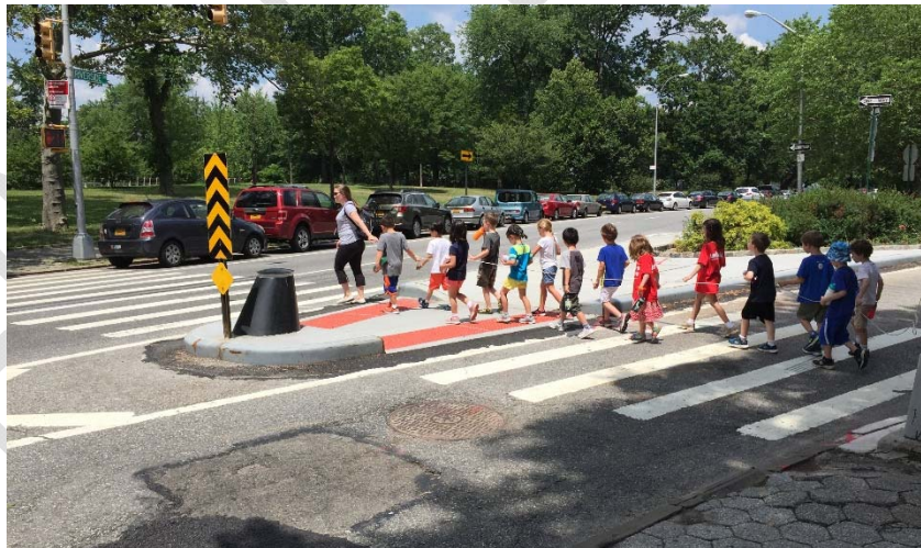
Example of a pedestrian refuge island in New York City. Source: New York City Street Design Manual.
