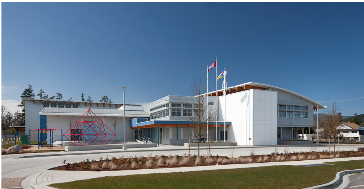
North Saanich Middle School, replacement school completed in 2012
