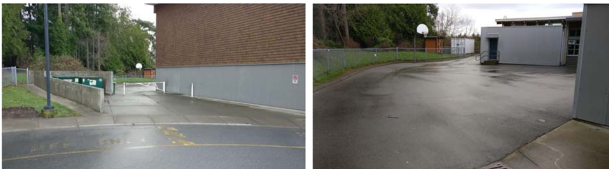
Figure 4: Western Paved Area (right) and Access (left)
